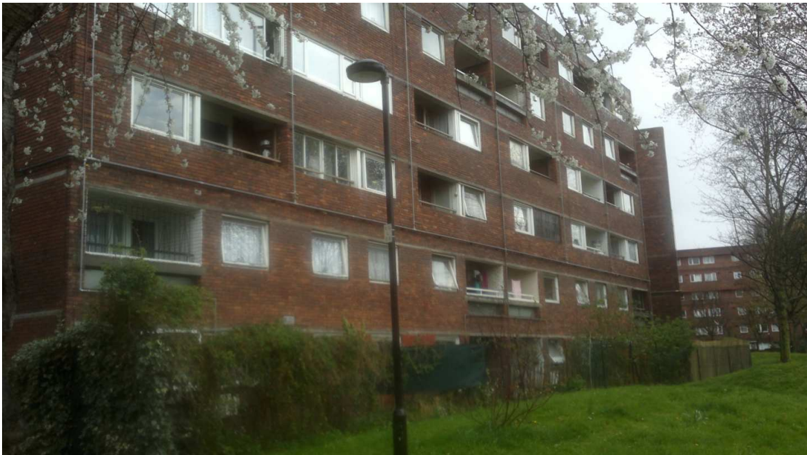
Photograph 1-showing Rhodeswell Road Block
